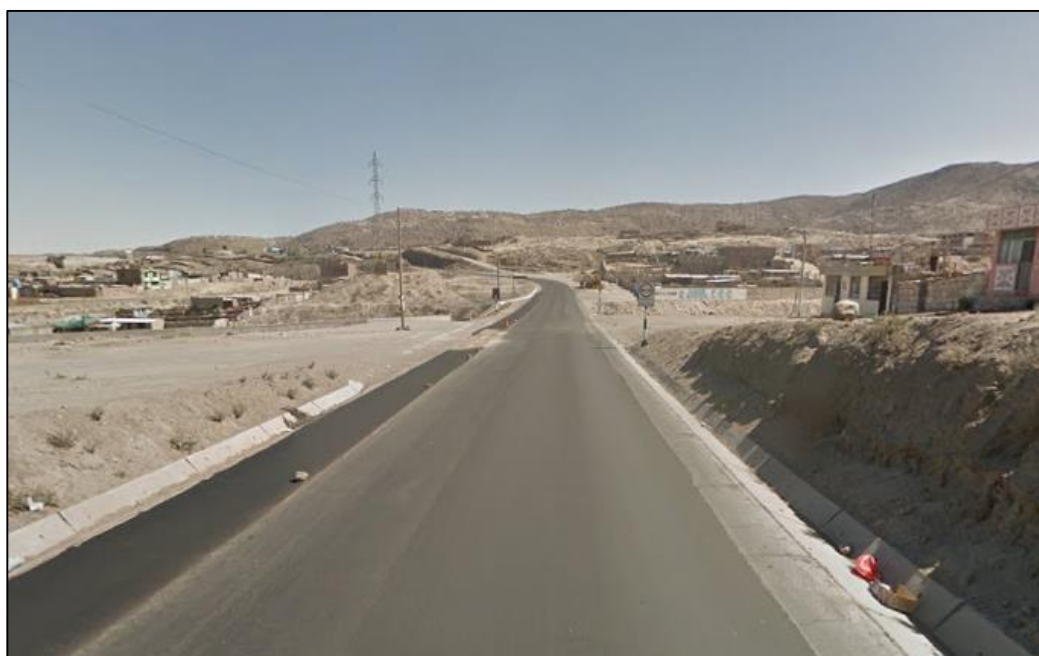
Figura 3-5: Carretera Arequipa – Yura (Tramo Final)
