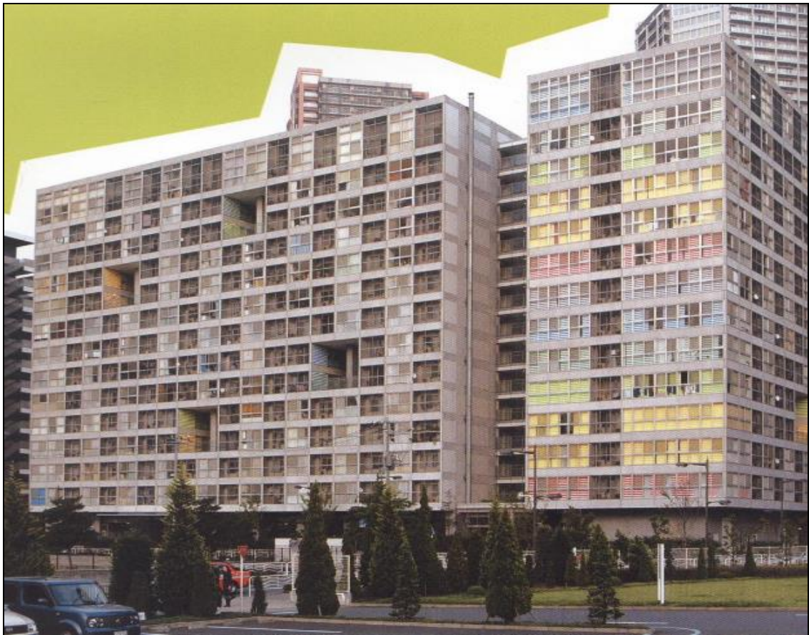
SHINONOME CANAL COURT
