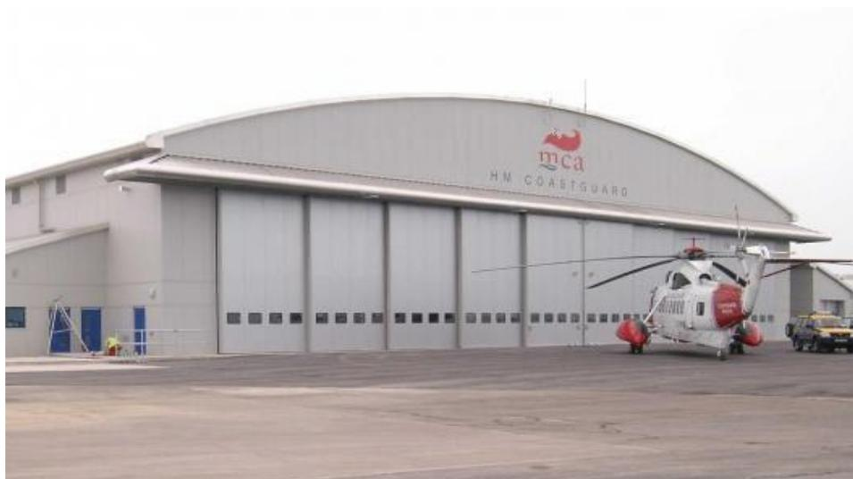
Figura 51. Puertas corredizas. Recuperado de [http://img.directindustry.es/images\\_di/photo-g/103929-9010535.jpg](http://img.directindustry.es/images_di/photo-g/103929-9010535.jpg)
