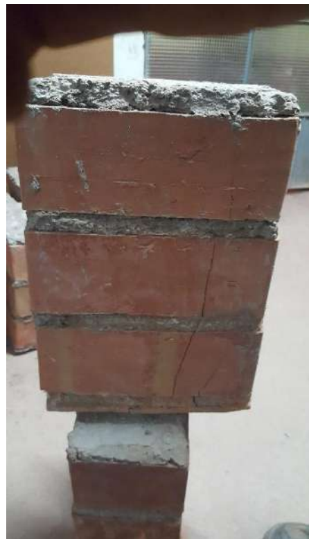
Presenta falla vertical
