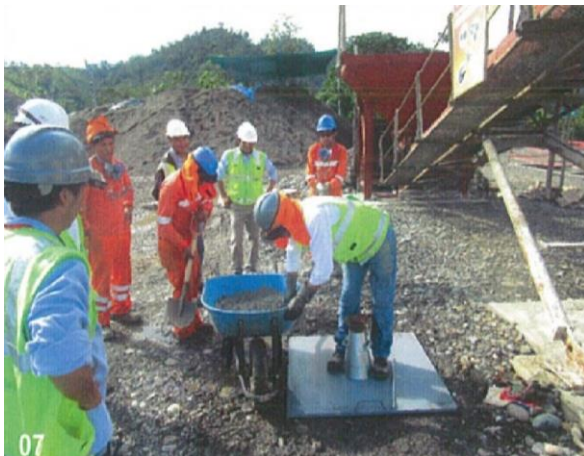
07 Control de slump.
