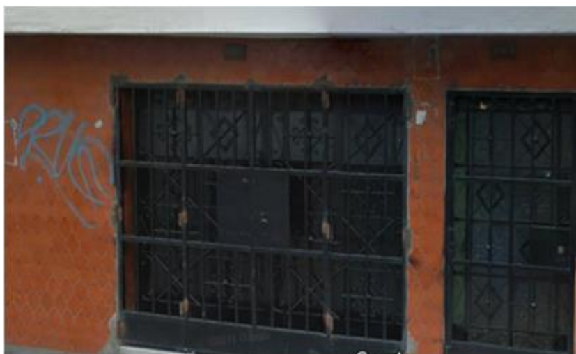
Local de RUBBER LINING PERU
