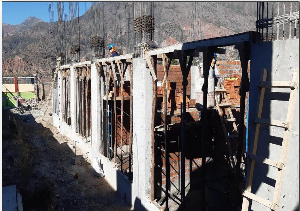
**FOTO 16: ARMADO DE ESTRUCTURAS – AMARRADO DE VIGAS A COLUMNAS**
