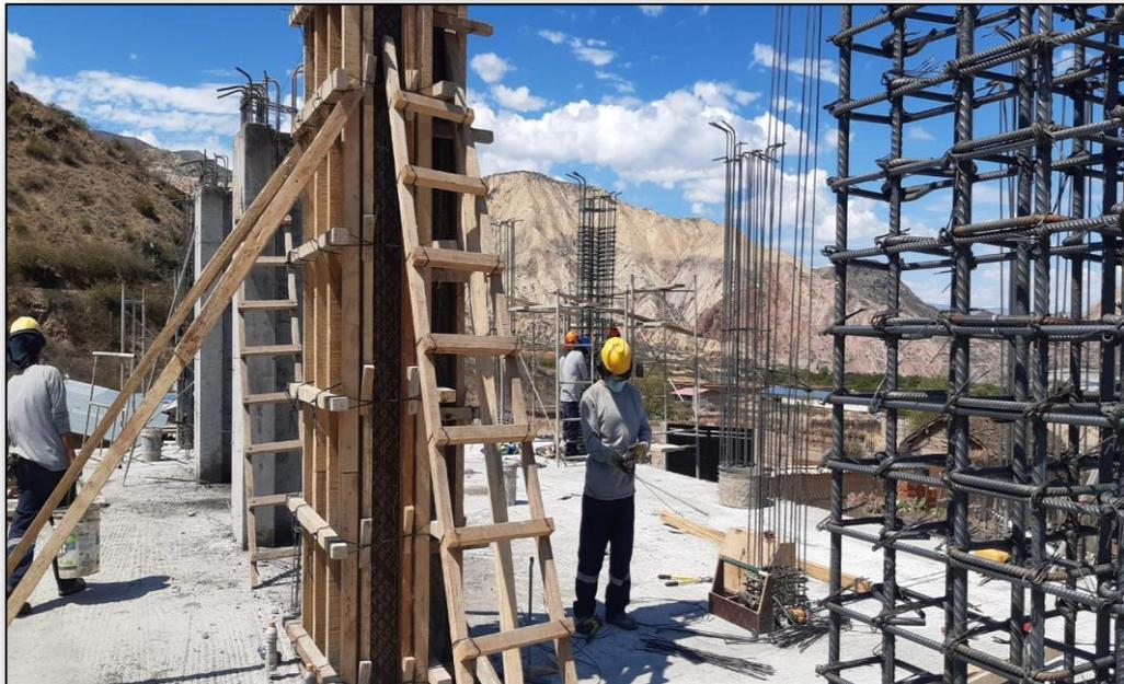
FOTO 22: VACIADO DE COLUMNAS CON CONCRETO 210 KG/CM2.
