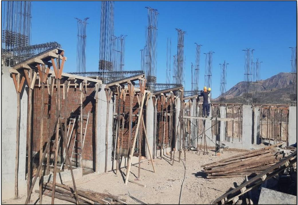
**FOTO 17: ARMADO DE ESTRUCTURAS – AMARRADO DE VIGAS A COLUMNAS**
