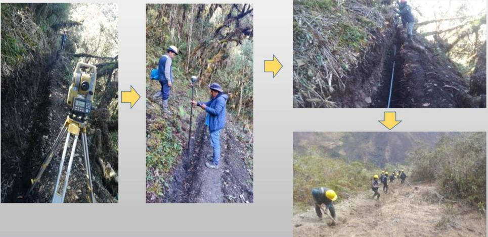
A sequence of four photographs illustrating the construction of a water line. The sequence starts with a surveying station, then workers measuring a path, then workers digging a trench, and finally workers laying a pipe.
