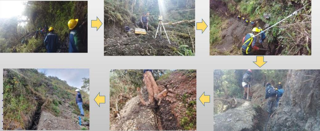
A sequence of six photographs illustrating the construction of a water line. The sequence starts with workers in a forest, moves to a surveying station, then to workers digging a trench, followed by workers laying a pipe, then workers clearing a path, and finally a completed trench.
