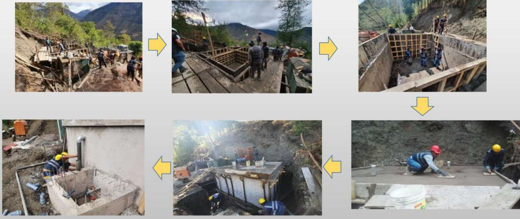
A sequence of six photographs showing the construction of a 15m3 reservoir. The images are arranged in two rows of three, connected by yellow arrows. The top row shows the initial site preparation and the construction of the concrete walls. The bottom row shows the completion of the walls and the final structure.
